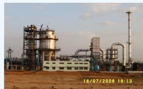
hazardous waste to the incinerator when operating conditions deviate from the design/acceptable range (Temp., residence time (RT), Turbulence)
